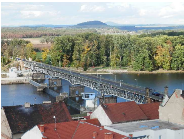
Fig. 5. Current view of the road bridge with the bridge locks (author's photo).
